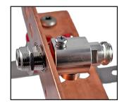
2. Install the surge protector into the ground bar. Place the ground bar between the rubber O-ring and lock washer.
